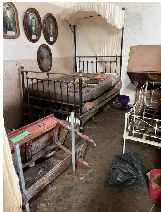
Flood damaged interior of museum – tide line evident
