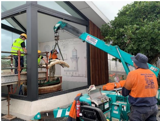
Reassembly in progress (Image: ICS)
