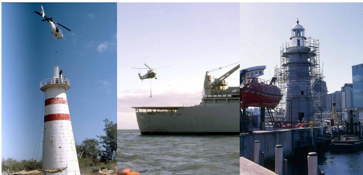
Cape Bowling Green lighthouse: disassembly, transportation and reassembly. Images: Ove Arup
