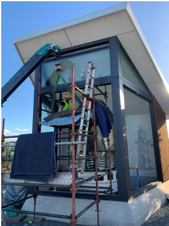
Reassembly in progress (Image: ICS)
