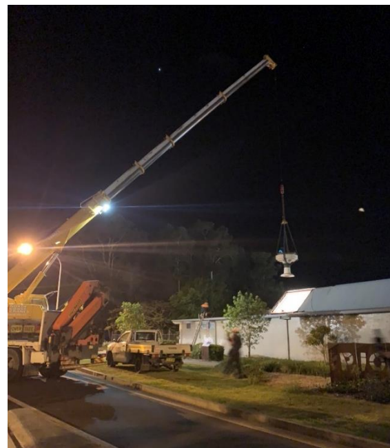
Lifting cast-iron pedestal through roof of old building (Image: ICS)
