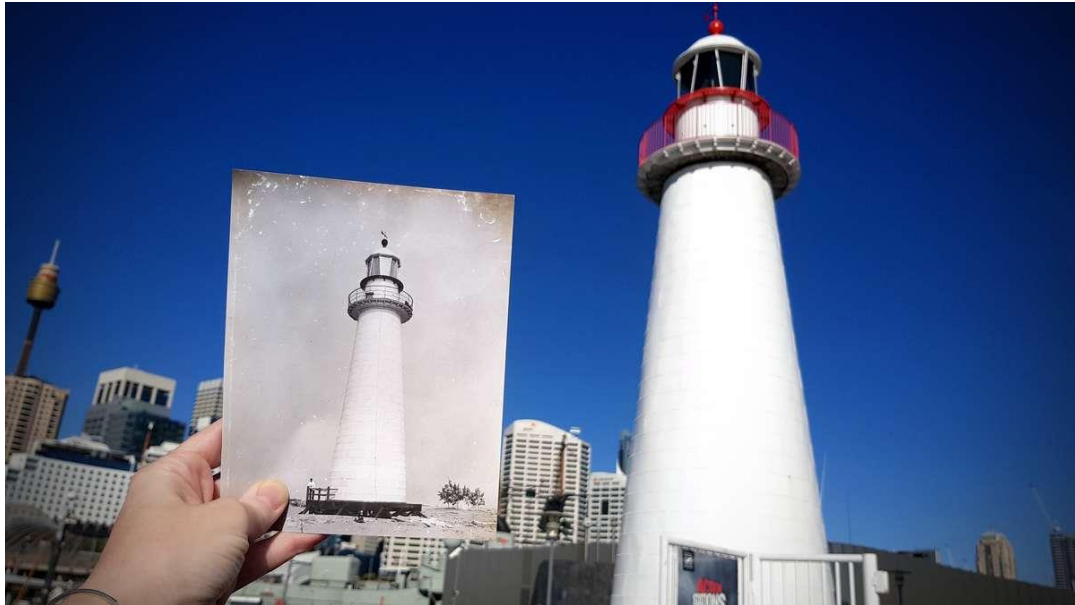
Cape Bowling Green lighthouse: disassembly, transportation and reassembly. Images: Ove Arup
