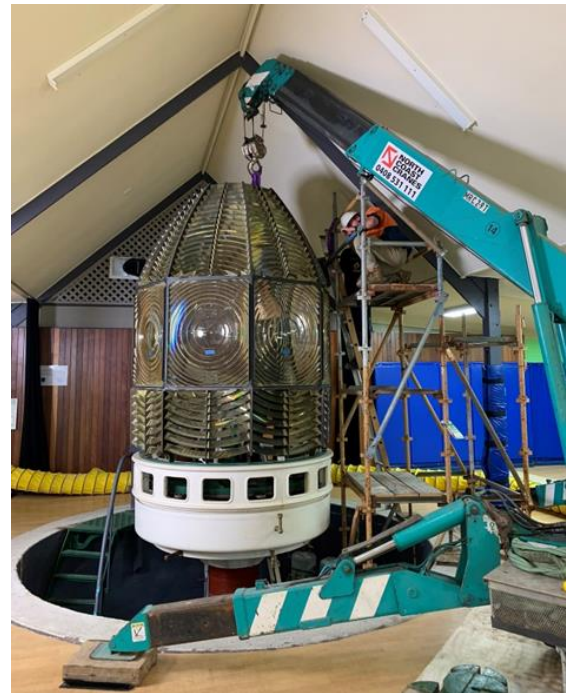
Commencing disassembly of SSILO (Image: ICS)
