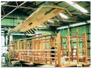
Restoration at Pichi Richi, South Australia—refitting the roof to Car No. 90, after body repairs. *Photograph courtesy of Carl Cedarblad*
