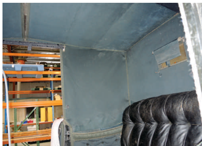
Landau interior after treatment - proper upper rear corner (area most visible during exhibition)
