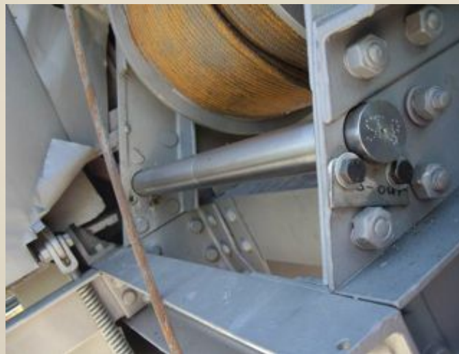
Figure 5 | Cable drums with missing jib pins before treatment (top) and with new stainless steel jib pins installed after treatment (bottom – note jibs not yet installed pending relocation for display).
