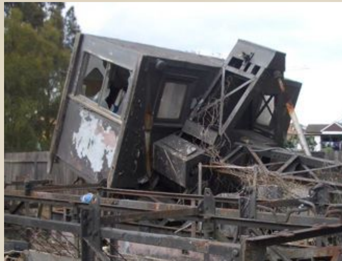
Figure 2 | Condition of crane before treatment.
