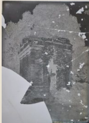
Figure 16 | Broken plate with missing glass and emulsion loss.
