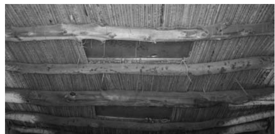
Figure 9: The construction of the roof with acacia beams and palm nerves
