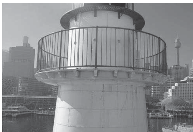
Corrosion stains down exterior of tower 2011.
