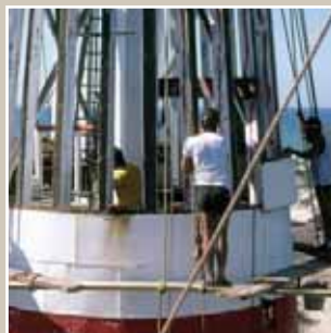
Work on the lighthouse at Darling Harbour
