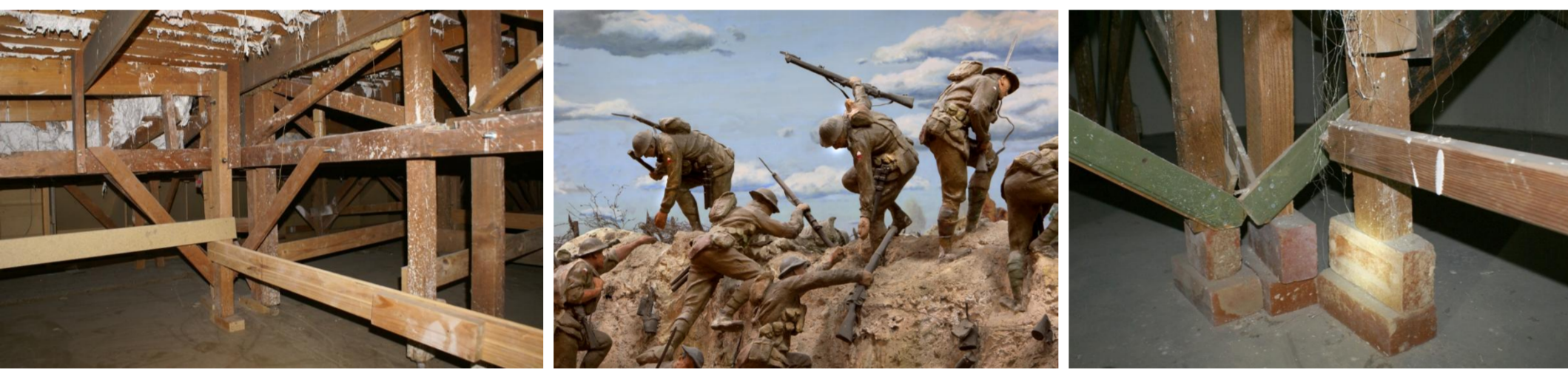
Mont St Quentin - plaster and lathe sections from below; detail of figures; Bullecourt - previously 'propped up' on bricks
