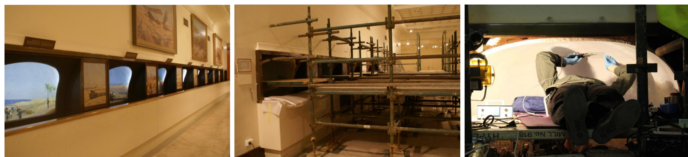
Transportation Series and façade - whilst gallery open; insitu scaffolding; Jocelyn in working position for consolidating flaking paint on backdrop
