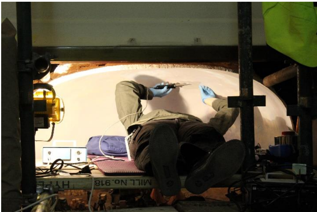
Jocelyn Evans activating the adhesive and repositioning the paint flakes with a heated spatula
