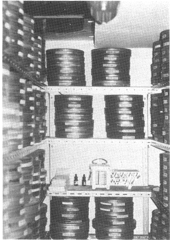
Figure 4. Interior of nitrate vault at the National Film Archive installation at Aston Clinton, outside London. Designed to hold 500 1000-foot cans on simple metal racking. The pressure vent is visible on the top left hand side.
