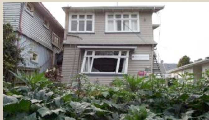
Figure 3 | Aftermath of the earthquake.
