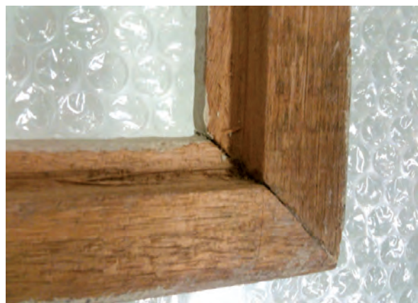
Figure 6. Detail of frame rebate for Mallee Switchbacks .
