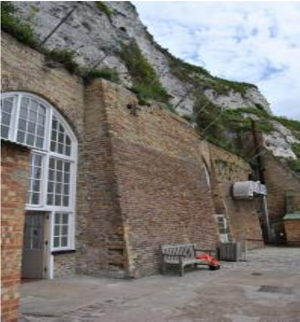
Secret War Tunnels at Dover. English Heritage
