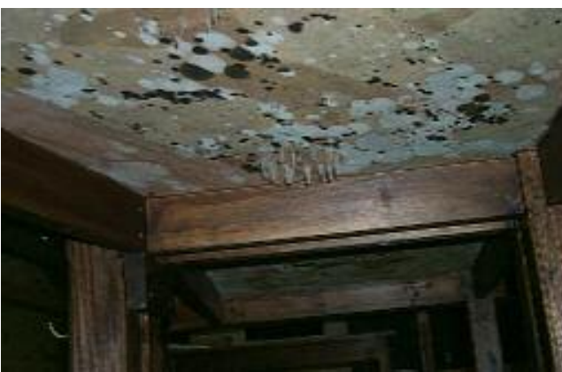
Underside of operations table. War Tunnels, Dover.
