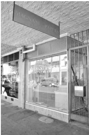
Figure 5: The original shopfront of Magnani Papers Australia in Smith Street Fitzroy, photographed in 2008
