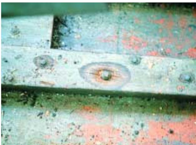
The bolts are corroding in high relative humidity conditions. The corrosion products are staining the wood, and will eventually cause splitting.
